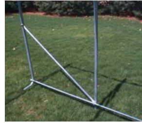
Structural wind brace on each corner
