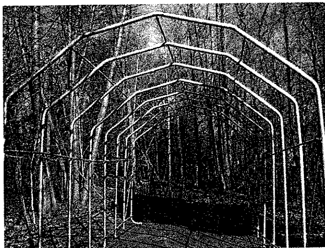
Add Cross Rails in preparation for adding Arch Assemblies
