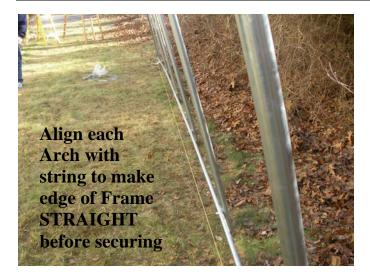
**Step 8**. Once frame is square and properly supported, tighten carriage bolts on all frame members, except for End Arch members to Cross Rails along base, side, and top. Support End Arch feet with patio blocks or bricks as needed if ground is soft and will not support weight well. After hardware is tightened, insert plastic end plugs 1-5/8" EP-1000 & 1" EP-1001 into all open ends of frame members.
