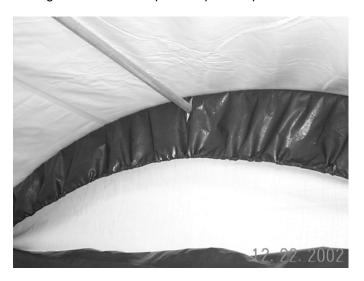
The rope slot should be located inside the unit, with the frame members passing through the pre-cut slots in the end panel/door. Replace the carriage bolts after putting the end panels into position.
