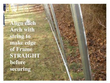
**Step 8**. Once frame is square and properly supported, tighten carriage bolts on all frame members, except for End Arch members to Cross Rails along base, side, and top. Support End Arch feet with patio blocks or bricks as needed if ground is soft and will not support weight. After hardware is tightened, insert plastic end plugs #EP-1000 (1 5/8") & EP-1001 (1") into all open ends of frame members.
