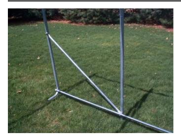
**Step 5**. Begin the Top Ridge Rail by placing the final ECR-2031 Plain End Cross Rail <u>underneath</u> the End Arch Tube. Secure the Cross Rail loosely with a Carriage Bolt CBN-3005-3 with washer and nut facing the interior of the unit. This begins the Top Ridge Rail. The other end of the Cross Rail goes on to of the Interior Arch as shown in the illustration above.
