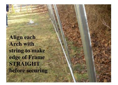
**Step 8**. Once frame is square and properly supported, tighten carriage bolts on all frame members, except for End Arch members to Cross Rails along base, side, and top. After hardware is tightened, insert plastic end plugs #EP-1000 (1 5/8") & EP-1001 (1") into all open ends of frame members.
