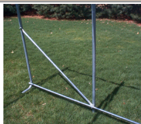
Structural wind brace on each side
