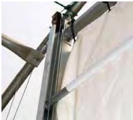
Door Tubes Inserted Into Door Track
