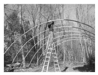
Interior Arch Assembly #5 and #6 have plain feet ends. The last Arch #7 will be the remaining End Arch Assembly with feet. Make certain to install the Wind Braces between the End Arch Assembly (#7) and the
