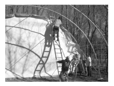
Adjust the door panel so that the edges do not come in contact with the ground. Cut the Slits as Needed To Adjust the Door Edge Off the Ground. Put an Electrical EMT or Pipe into the bottom edge to put weight on the door fabric.
