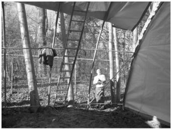
Pull Main Cover over frame with rope threaded through one of the grommets near the end flap. Be careful not to snag or rip the cover on any exposed bolts or rough ends.
