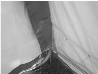
Inside Corner view showing Main Cover and End Panel Door properly laced and secured with turnbuckles.
