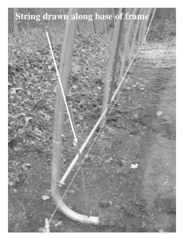
Measure the base span of each arch, side to side. The outside of the arch bases should be 30'. Too wide a span will weaken the frame resistance to load, such as snow, and prevent the doors and main cover from fitting properly. Adjust each arch to the correct width, using the first side aligned above.
