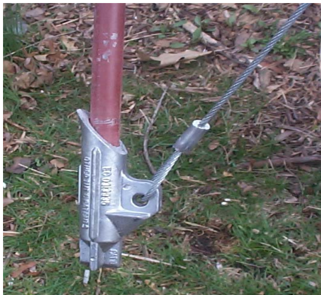
Drive Rod inserts into Anchor Head
