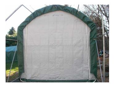
Note: After door panel is installed with all slack out of rope, adjust/snug the end panel by turning the turnbuckles or repeating step 3 on a regular basis
