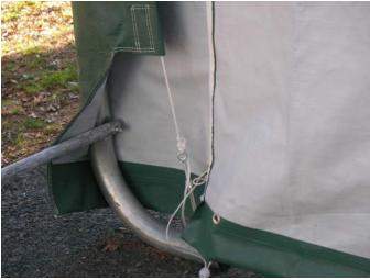
Door Turnbuckle Attached to Base Foot
