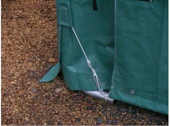
Main Cover Turnbuckle secured to Base Foot
