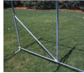
Structural wind brace on each side
