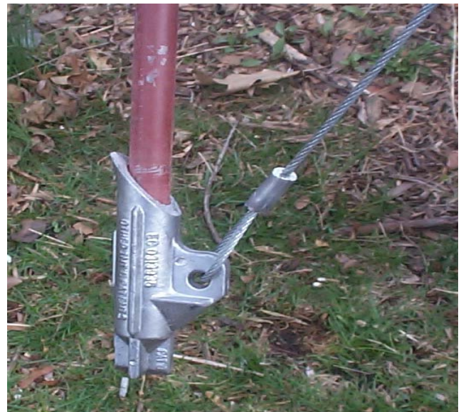
Drive Rod inserts into Anchor Head
